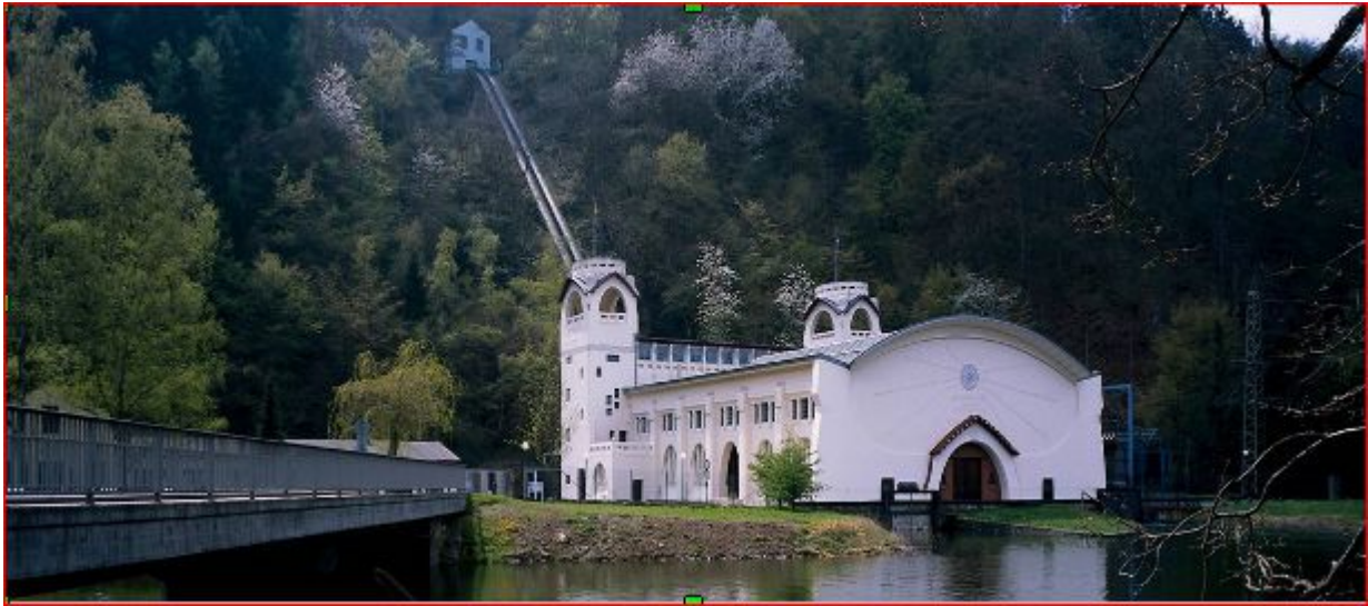
(Photo: Heimbach hydropower plant)
